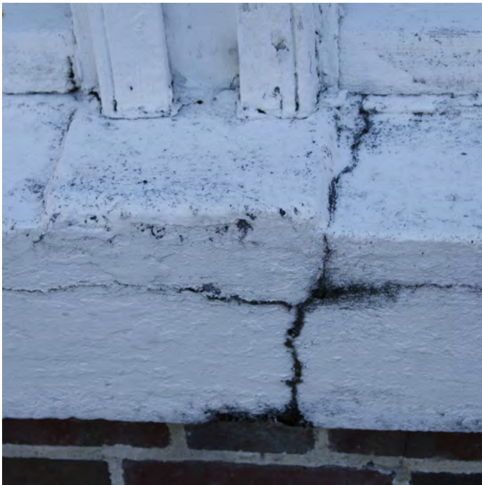
06 Existing condition of crack at window sill
