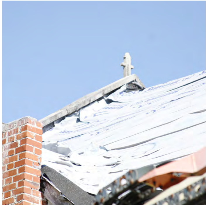
26 Existing conditions of partial roof and valley condition
