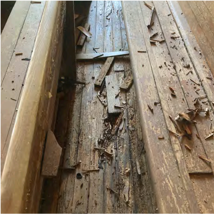
47 Existing condition of wood planks at second floor
