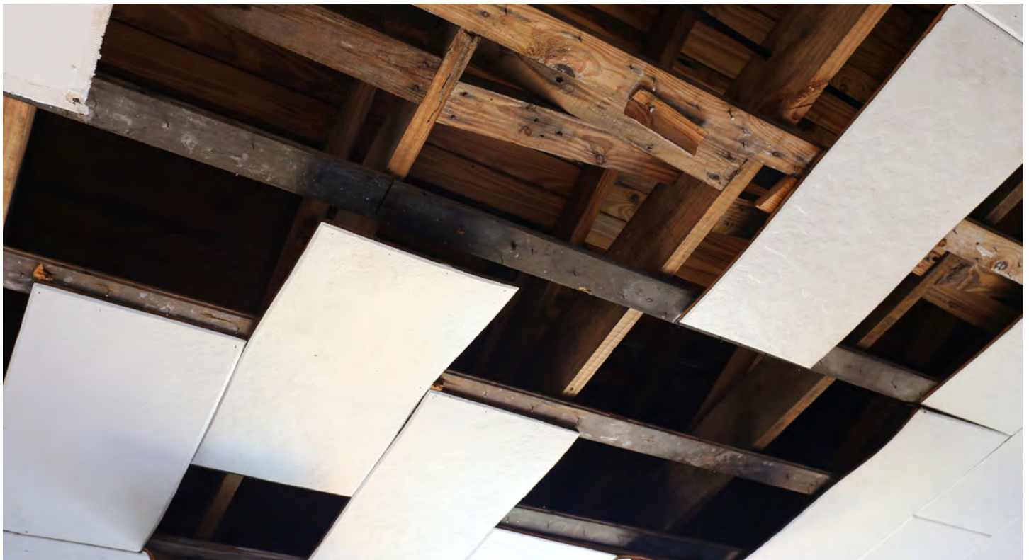
51 Existing condition of ceiling prior to partial removal of ceiling tiles
