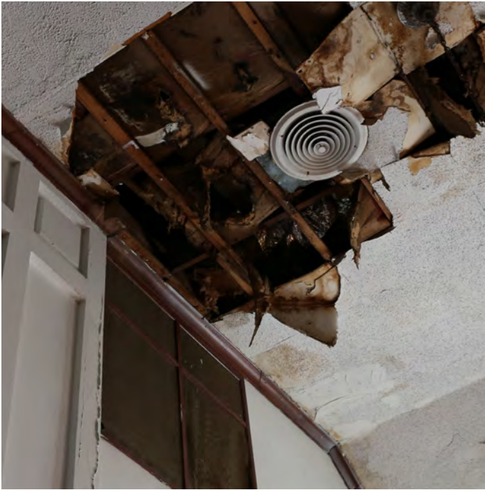
49 Existing condition of water damage at second floor ceiling
