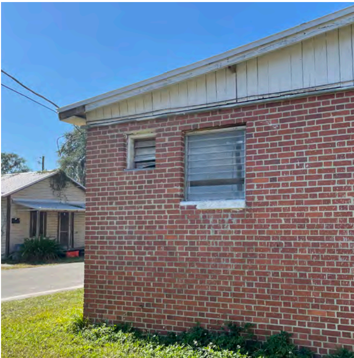
19 Southeast corner of add-on depicting existing fascia, vertical wood siding at roof, and lower window conditions
