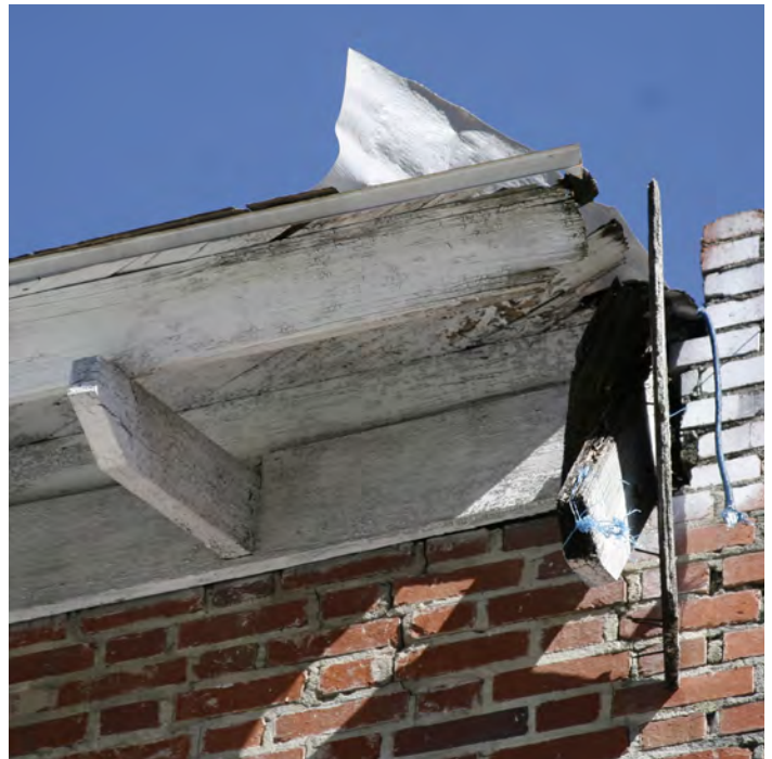
28 Existing conditions of roof soffit, fascia, and rafters
