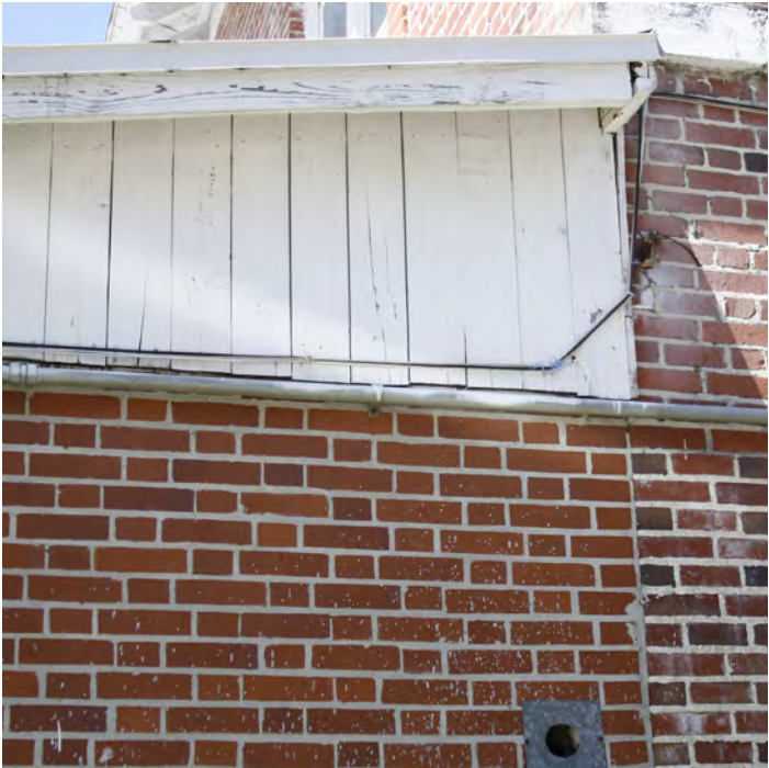
22 Existing condition of wood siding at roof at add-on
