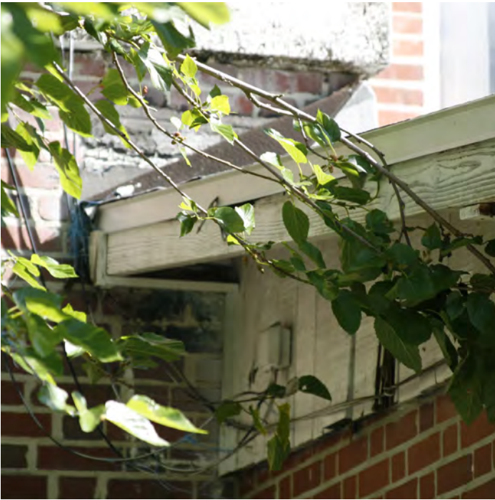
23 Partial south elevation of add-on depicting deterioration of existing fascia, soffit and existing conditions
