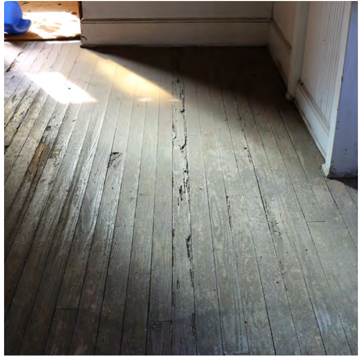
21 Existing condition of wood planks at upper lobby
