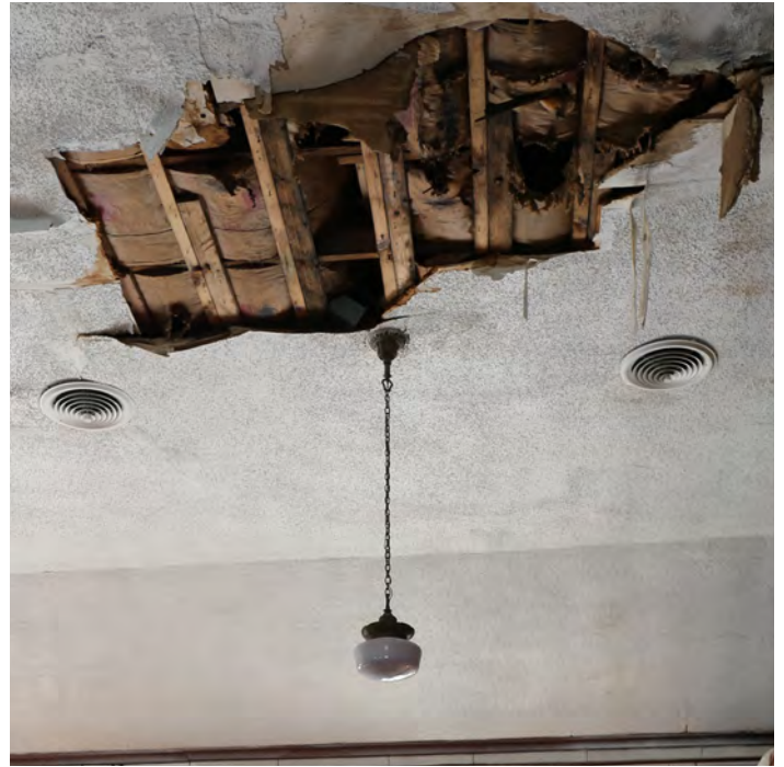
50 Existing condition of water damage at second floor ceiling
