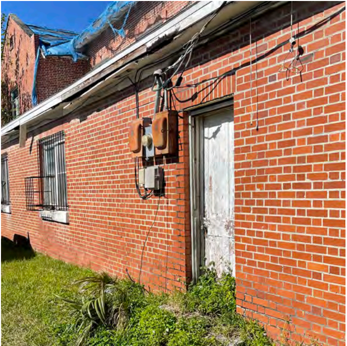
24 Partial south elevation of add-on depicting deterioration of existing fascia, soffit and existing conditions
