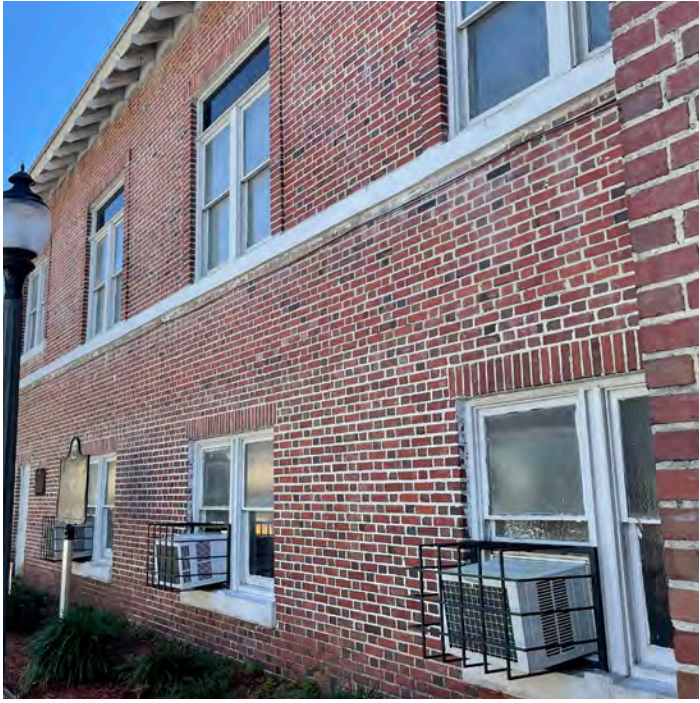
16 North elevation depicting existing historic brickwork, exterior windows and window A/C units
