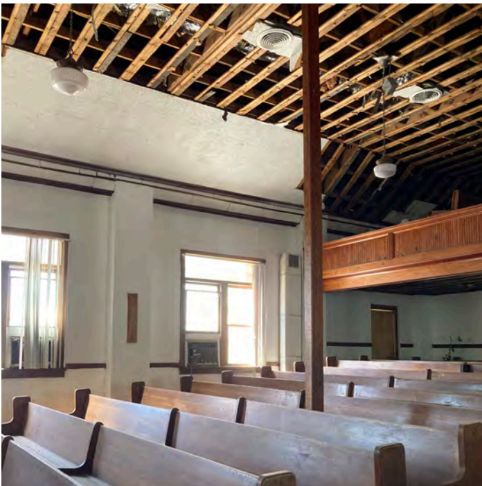
33 Existing condition of second floor interior including pews and ceiling after partial removal of ceiling tiles
